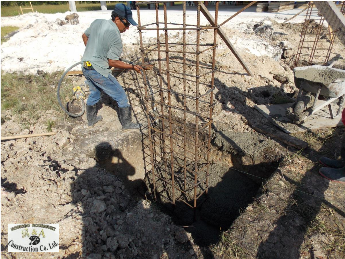
MUFFLES JUNIOR COLLEGE - METAL SHED & SHED EXTENTION - ORANGE WALK DISTRICT
