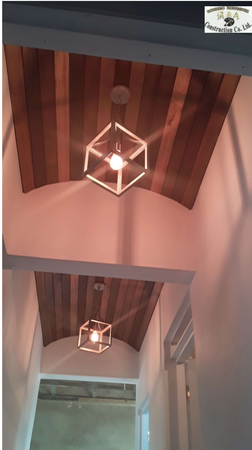
WOODEN DOME CEILING WORKS - FINCA SOLANA
