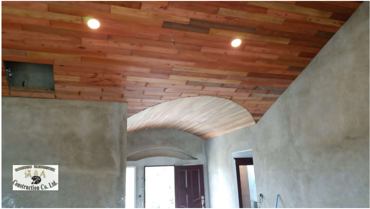
WOODEN CEILING WORKS - FINCA SOLANA
