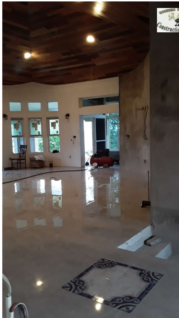
WOOD CEILING & FLOOR TILE WORKS - FINCA SOLANA
