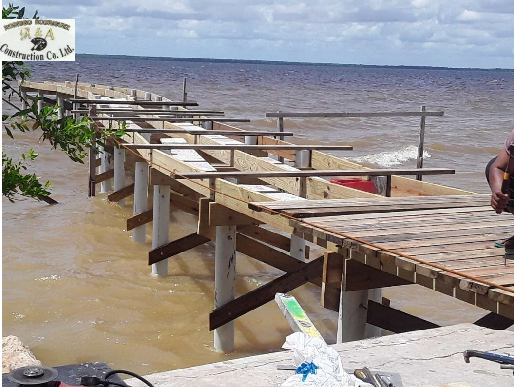
PIER CONSTRUCTION - FINCA SOLANA
