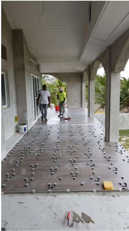
FLOOR TILE WORKS - FINCA SOLANA
