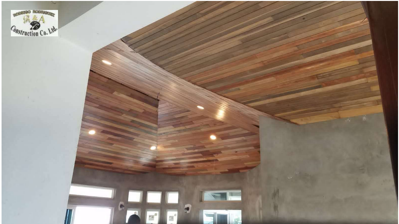
WOODEN CEILING WORKS - FINCA SOLANA
