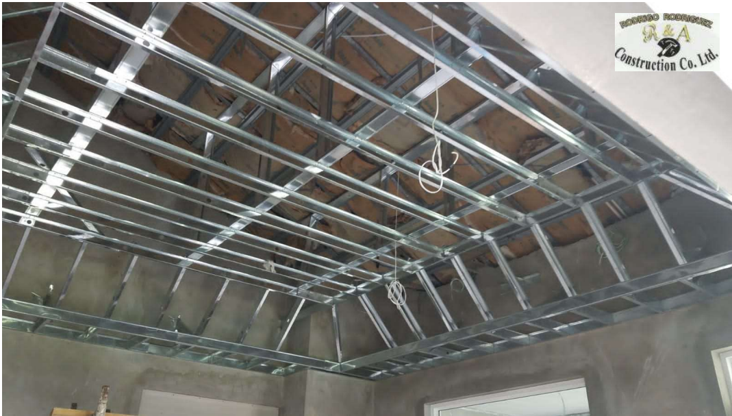
CEILING METAL FRAME WORKS - FINCA SOLANA
