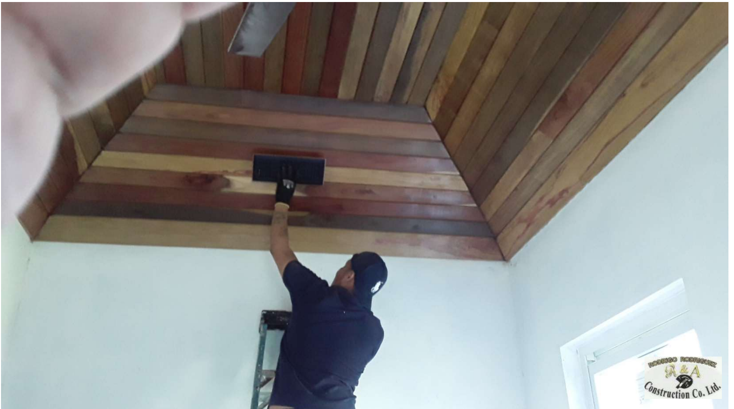
WOOD CEILING FINISH - FINCA SOLANA
