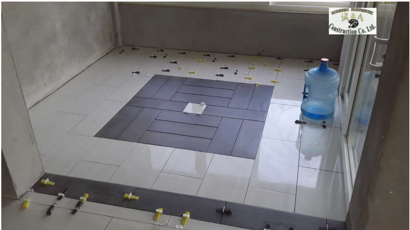
FLOOR TILE WORKS - FINCA SOLANA
