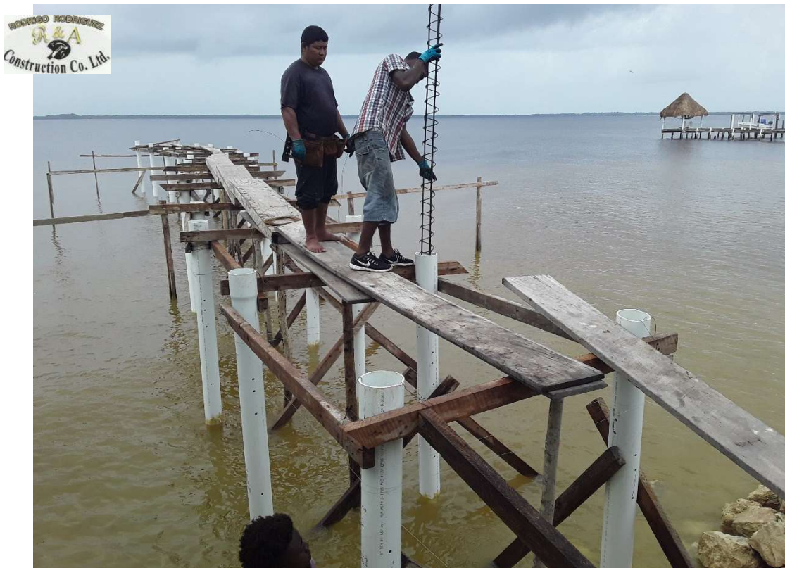
PIER CONSTRUCTION - FINCA SOLANA
