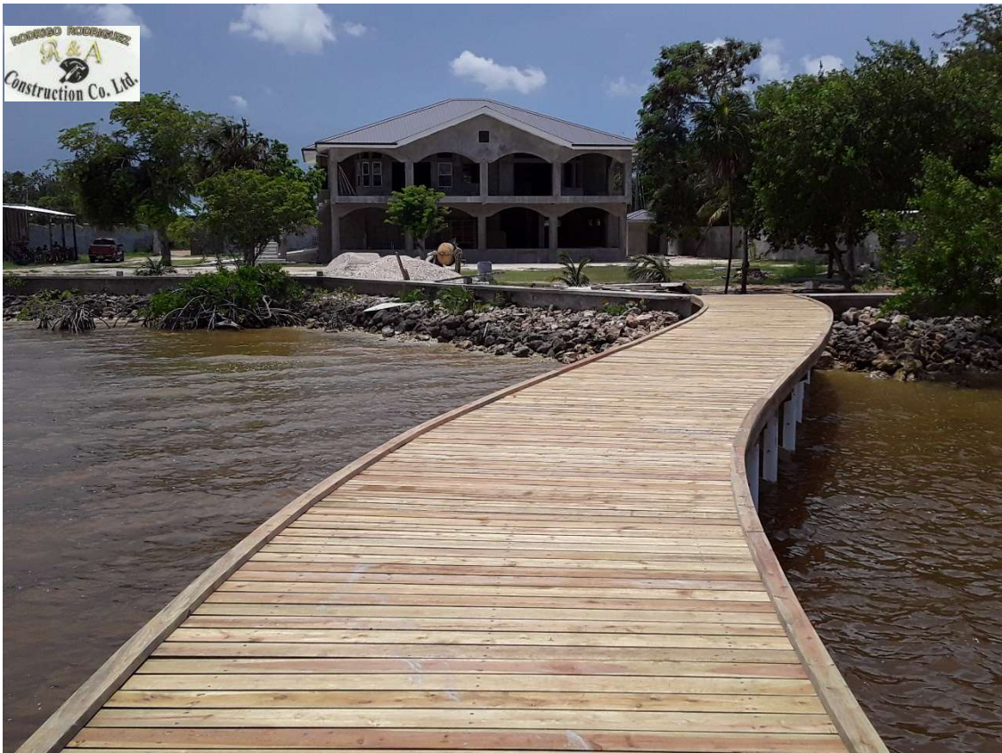
PIER CONSTRUCTION - FINCA SOLANA
