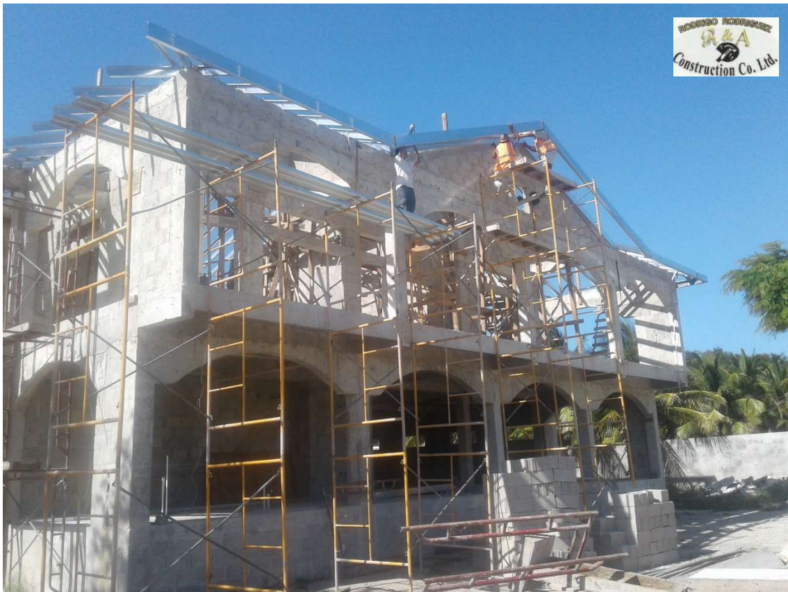
METAL ROOF FRAMING - FINCA SOLANA
