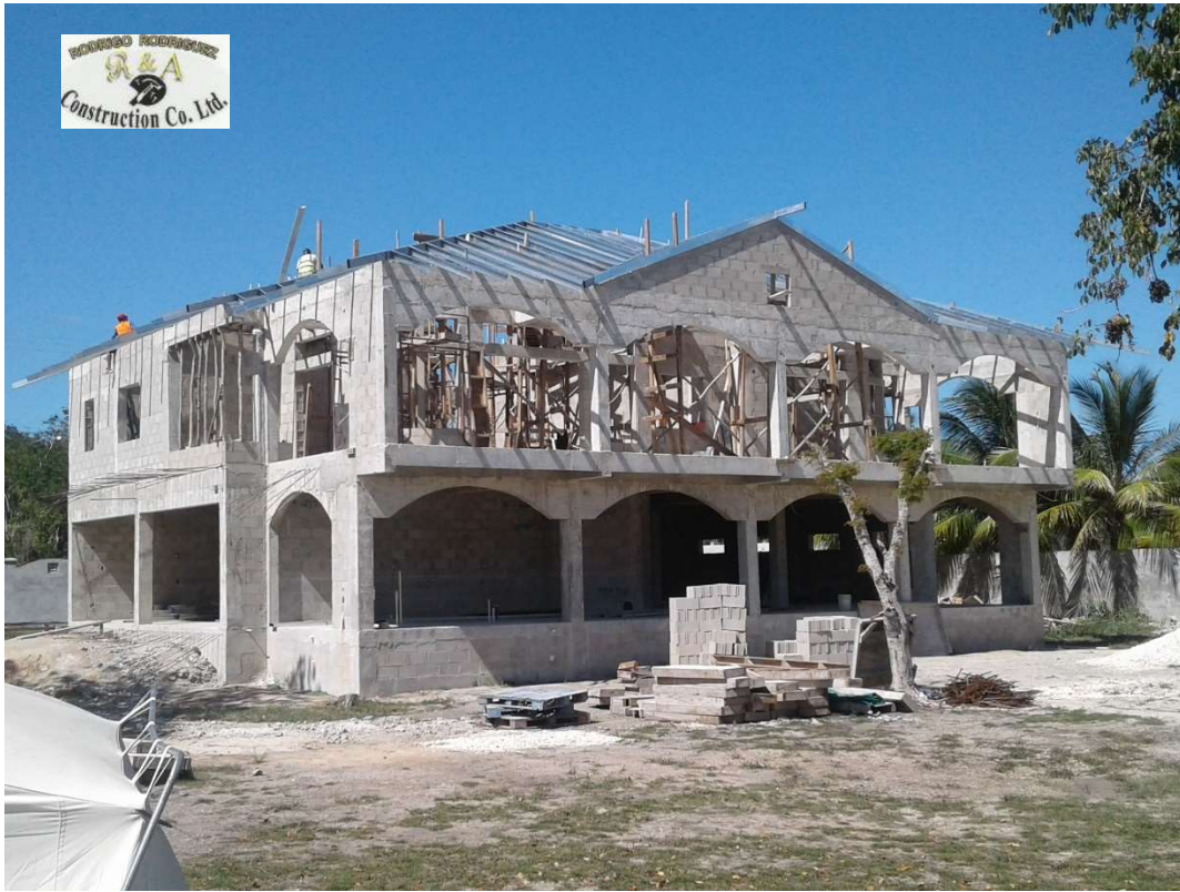
METAL ROOF FRAMING - FINCA SOLANA
