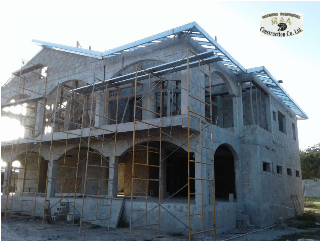
METAL ROOF FRAMING - FINCA SOLANA
