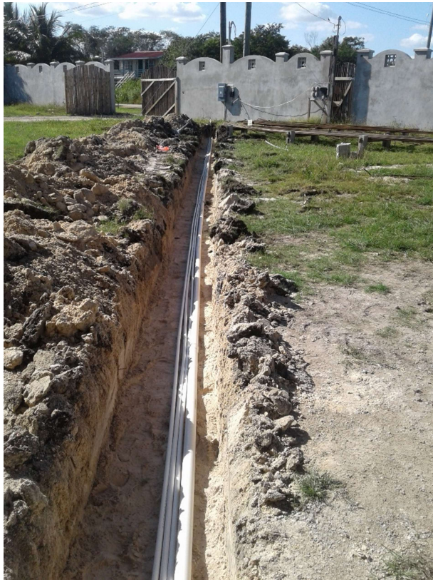
MAIN ELECTRICAL & DATA & CABLE LINES - FINCA SOLANA
