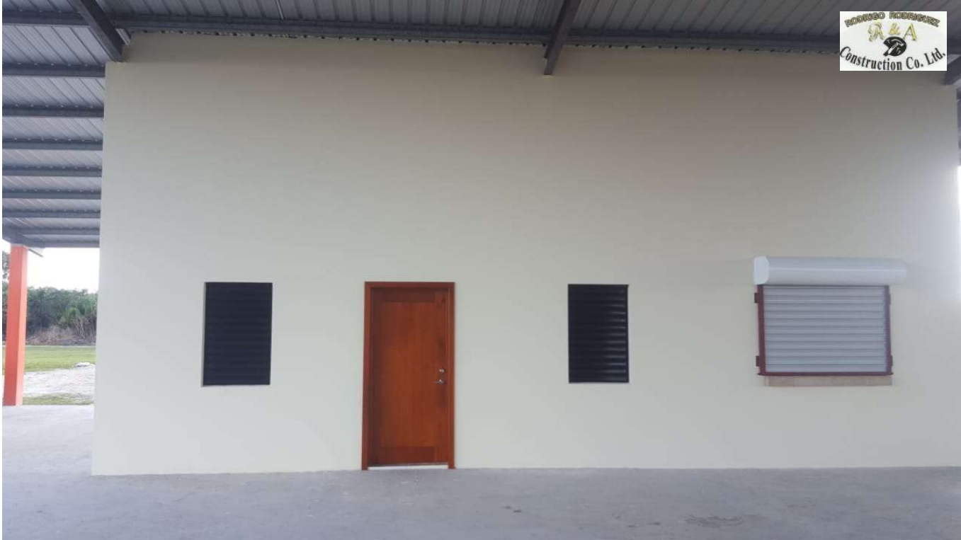
MUFFLES JUNIOR COLLEGE - CAFETERIA EXTERIOR - ORANGE WALK DISTRICT
