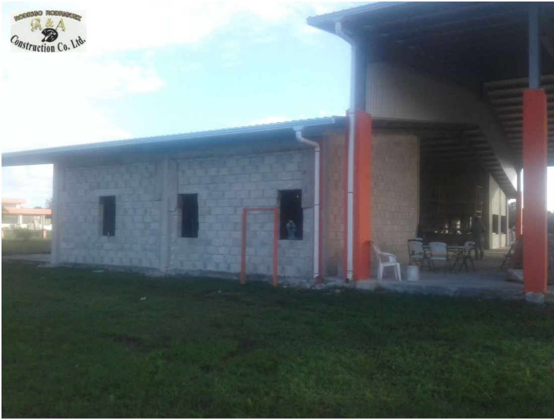
MUFFLES JUNIOR COLLEGE - CAFETERIA & STORE ROOM PROJECT - ORANGE WALK DISTRICT
