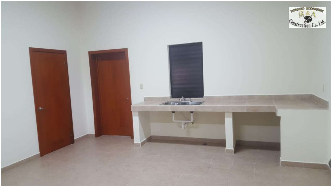
MUFFLES JUNIOR COLLEGE - CAFETERIA COUNTERS, WINDOWS, SHUTTERS & DOOR - ORANGE WALK DISTRICT
