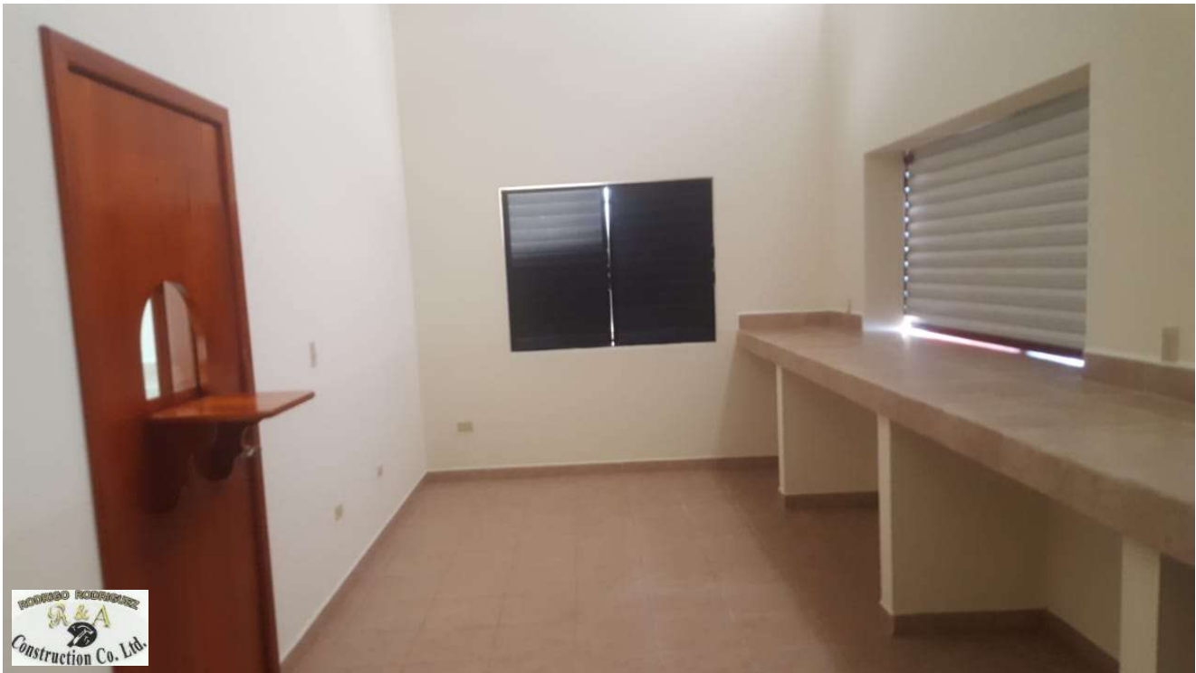
MUFFLES JUNIOR COLLEGE - CAFETERIA COUNTERS, WINDOWS, SHUTTERS & DOOR - ORANGE WALK DISTRICT
