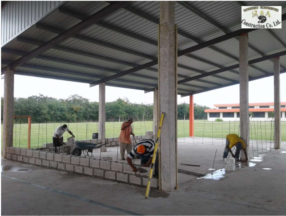
MUFFLES JUNIOR COLLEGE - STORE ROOM PROJECT - ORANGE WALK DISTRICT
